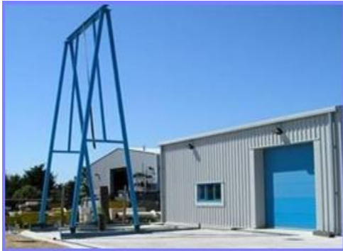
ALC's test rig at Great Yarmouth
